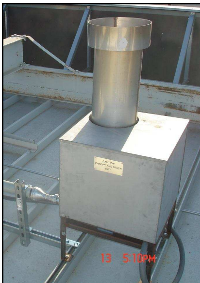
Processor mounted on canopy with optional 5" Legs
